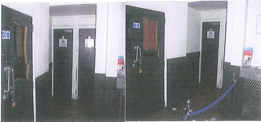
Entry Area to Male and Female Customer Toilets
