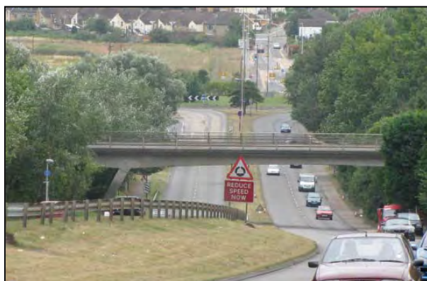
Figure 5.7: Upchat Road bridge
