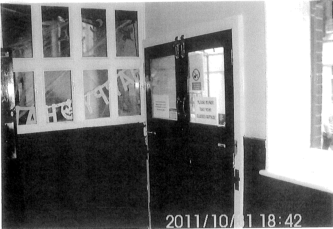
Entrance doors to the basement bar stairwell.
