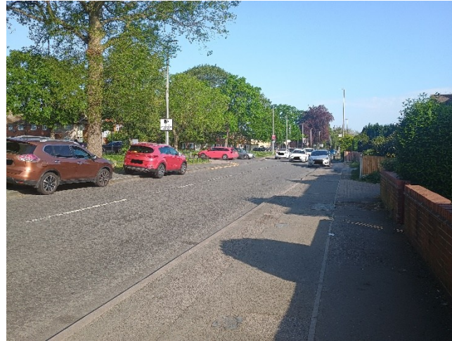
Pavement parking on Walderslade Road (facing North)
