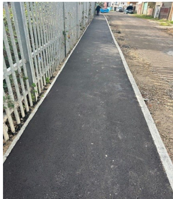
Granville Road, Gillingham (rear) - After
