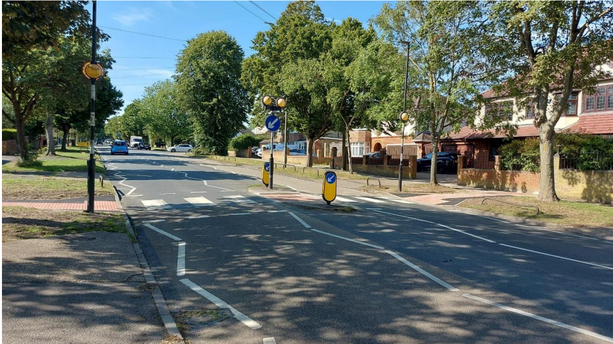
Figure 4. Crossing upgrade – City Way (Rochester)
