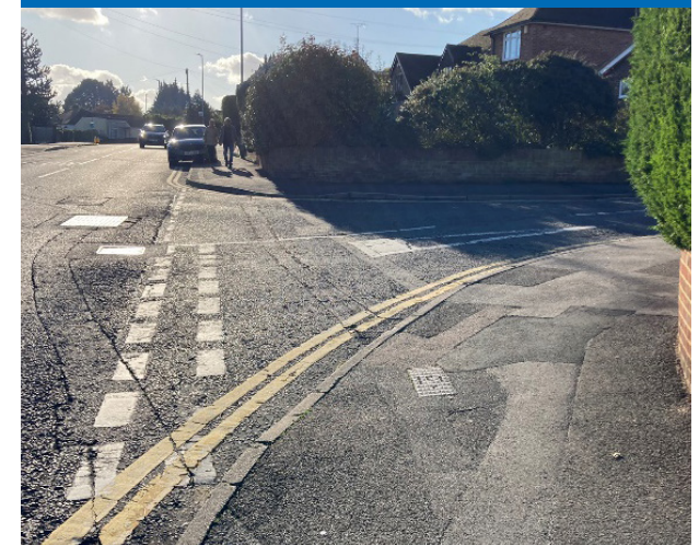
Wide junction with no tactiles or dropped kerbs
