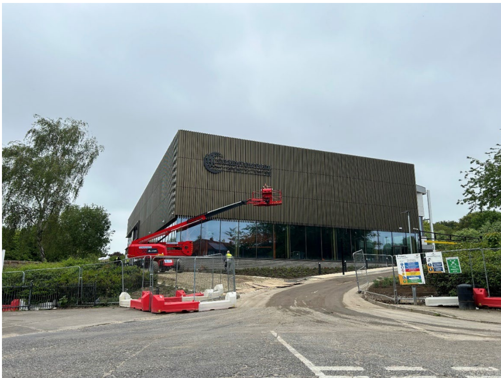
Construction at Cozenton Park Rainham nearing completion
