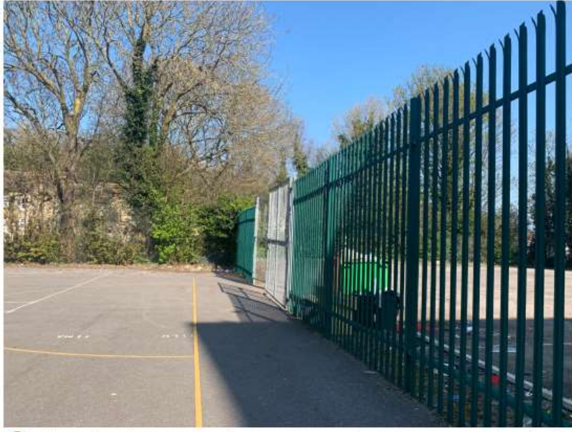
V2 View of gate separating hard sports area from the grass playing fields
