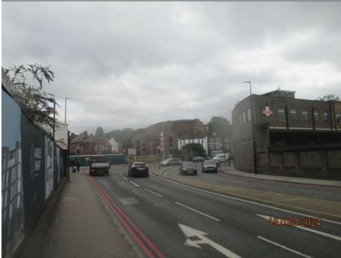
Now – Buildings onsite demolished
