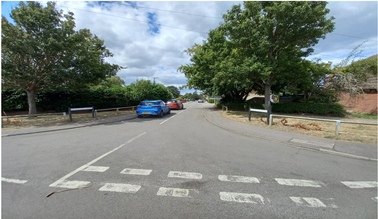
Wider View of Junction Coronation Road/Edinburgh Road
