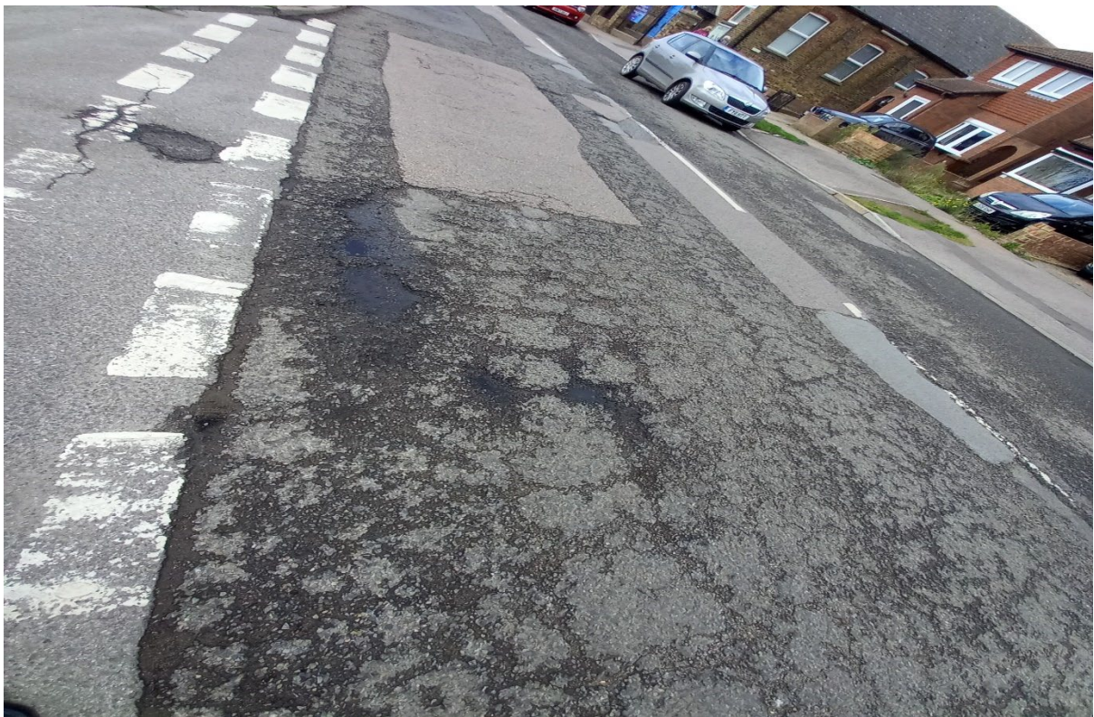
Road Surface Junction Chapel Road with Coronation Road
