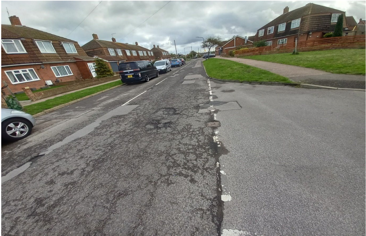
Road Surface Junction Chapel Road with Coronation Road
