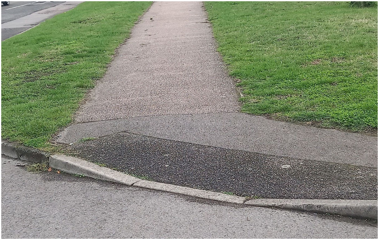
Drop Kerb Junction Chapel Road/Coronation Road
