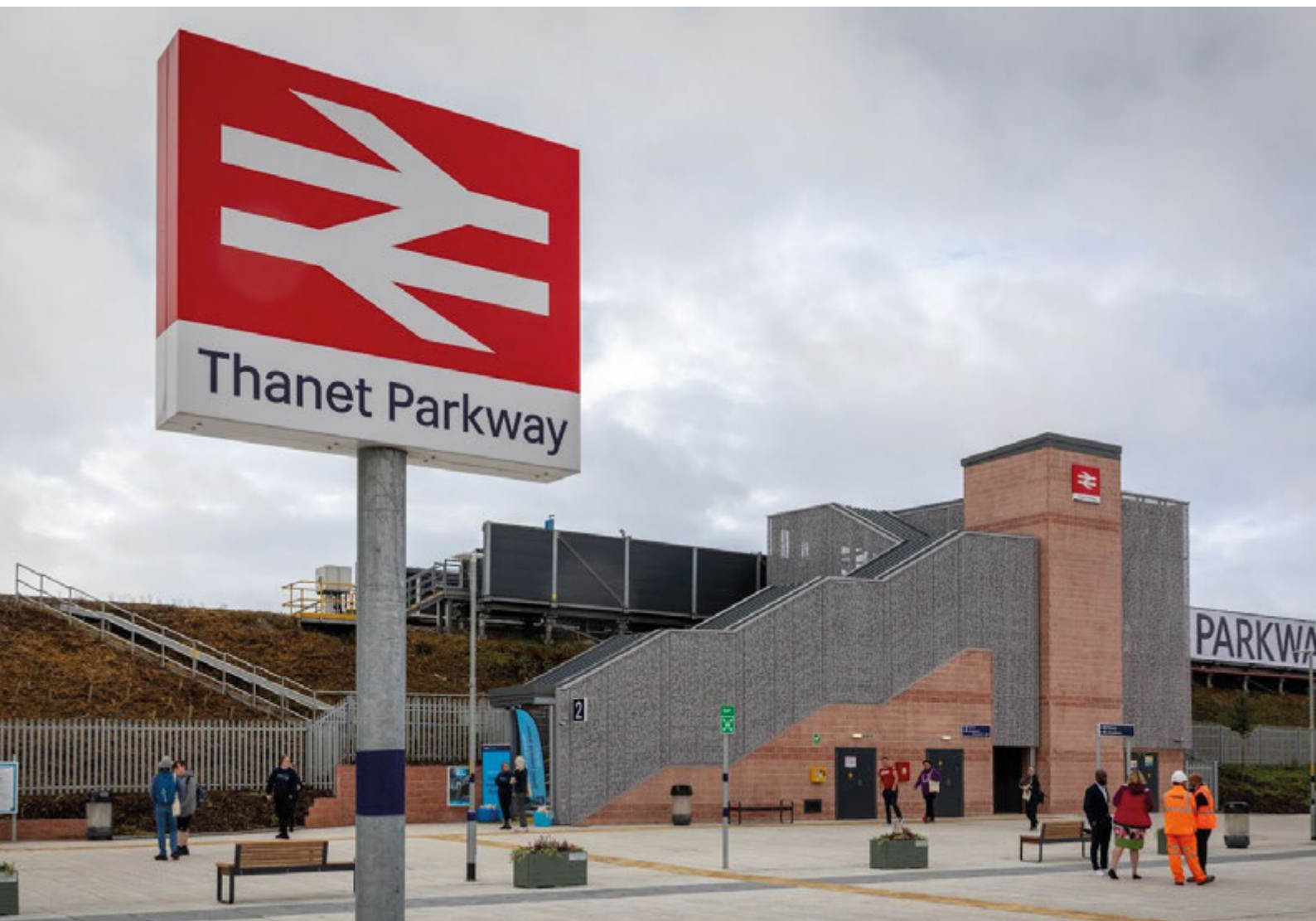
Thanet Parkway rail station.
