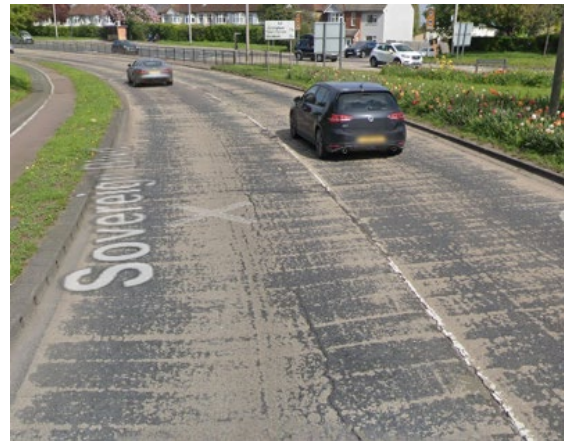
Watling Street, Gillingham (before)
