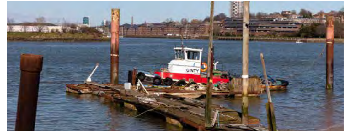
Existing small timber jetties leading to boat activities
