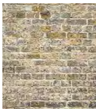
Buff brick walls
