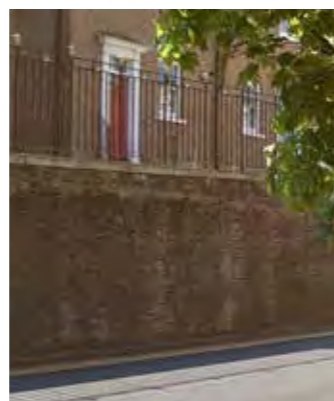
Brick wall and metal railing
