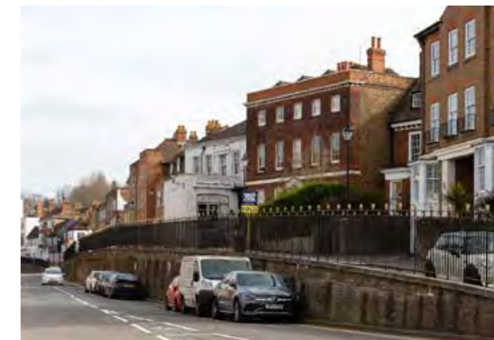
Height difference across the High Street which creates issues with permeability and access.
