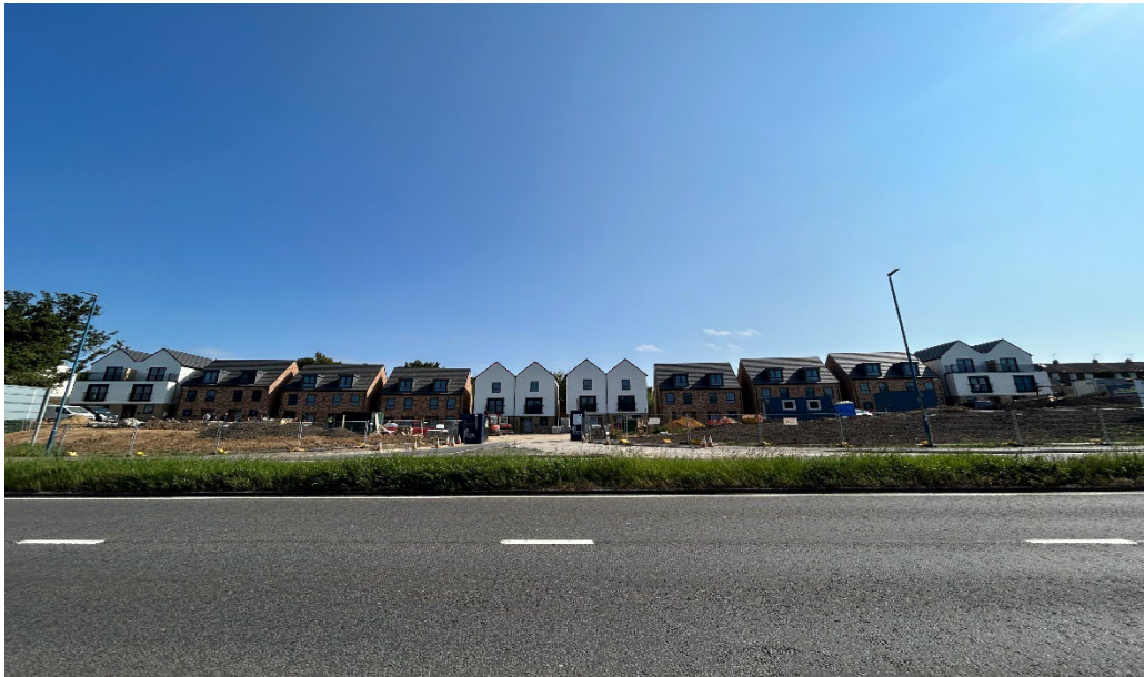
Affordable housing scheme Gillingham
