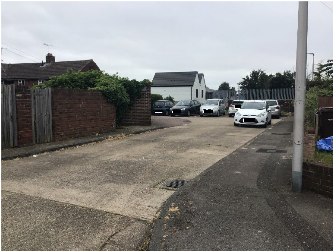
Photo 5: Eastern end of close, with four more garages which could if removed free up parking for all residents
