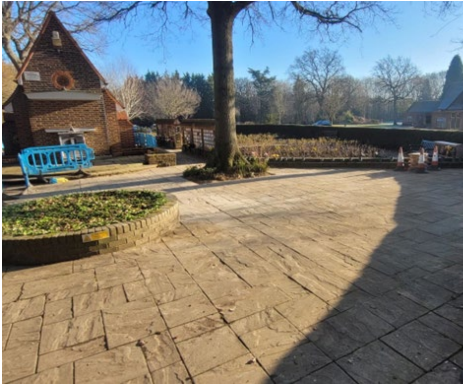
Photo of footpaths improvements behind the Chapel of Meditation (Crematorium)
