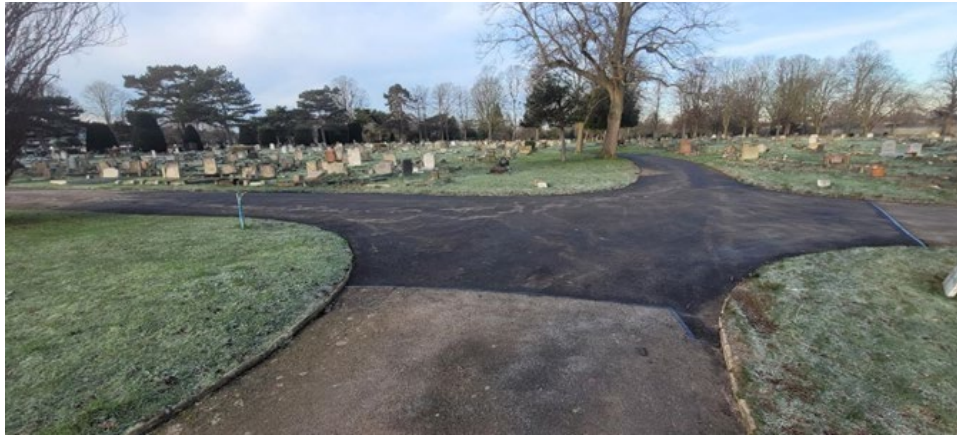
Photo of Woodlands Cemetery showing highway improvements
