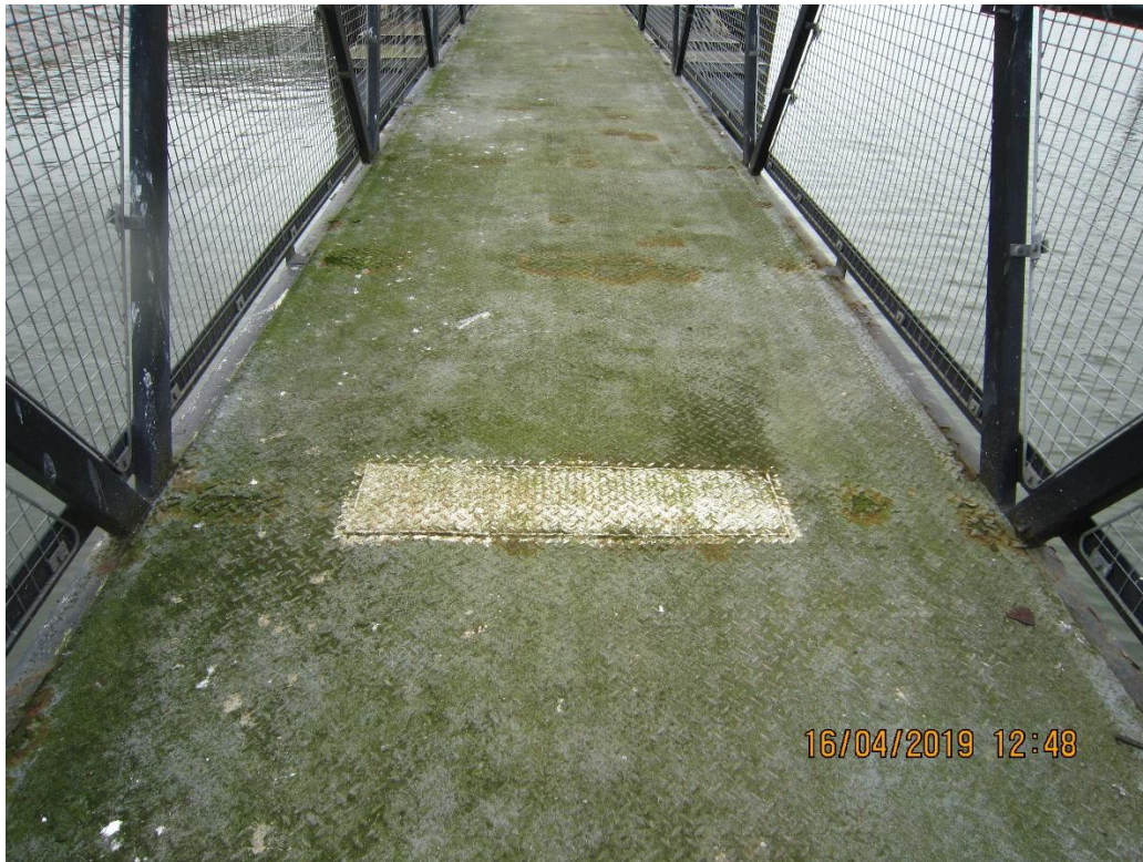
Cut out and plated over.
