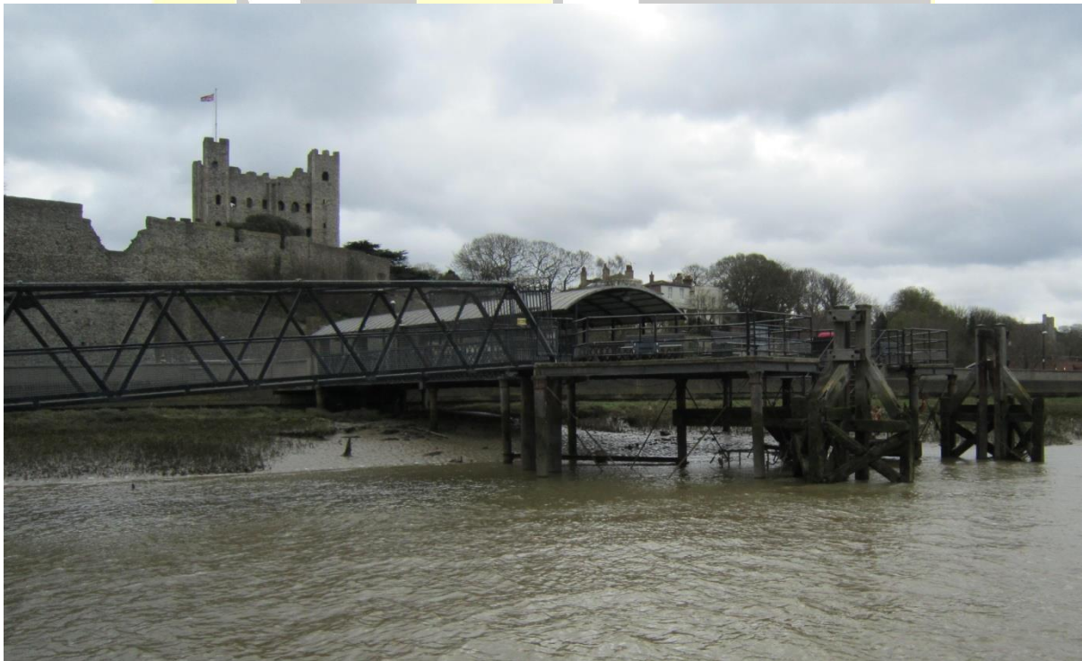
Condition of jetty structure, pontoon and Brows
