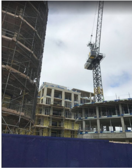
Construction works at Chatham Waterfront
