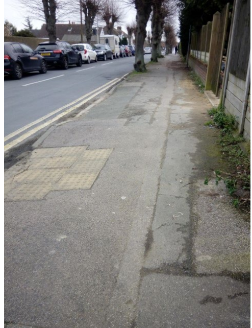
Thames Avenue, Rainham (Before)
