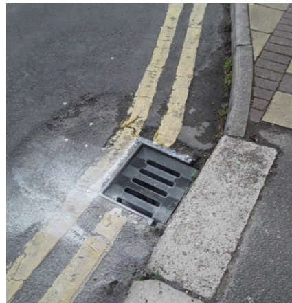
Composite cover fitted as result of emergency
