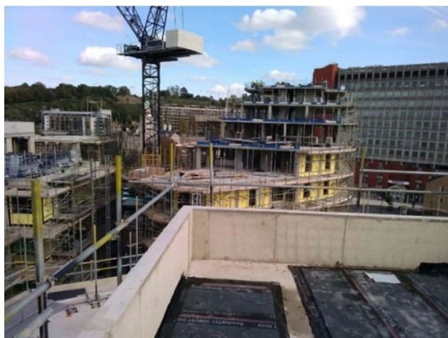
Photograph, showing concrete frame complete to top of Block C
