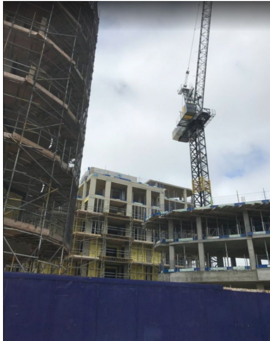
Construction works at Chatham Waterfront
