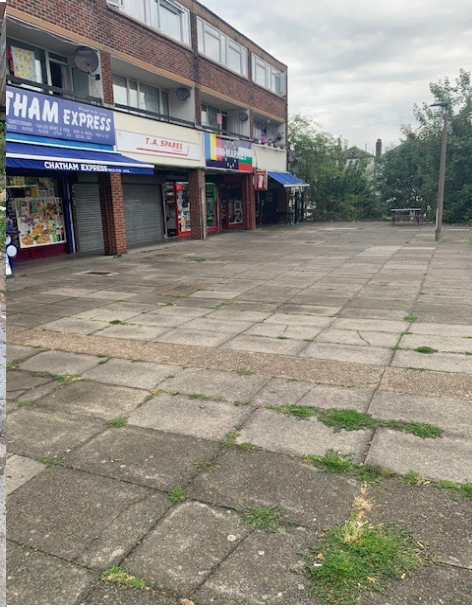
Area in front of Ordnance Street shops
