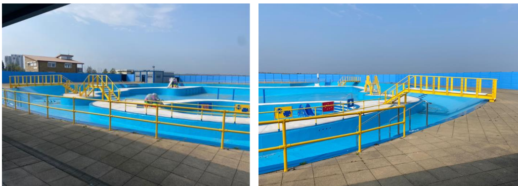
The Strand Pool Following Repaint
