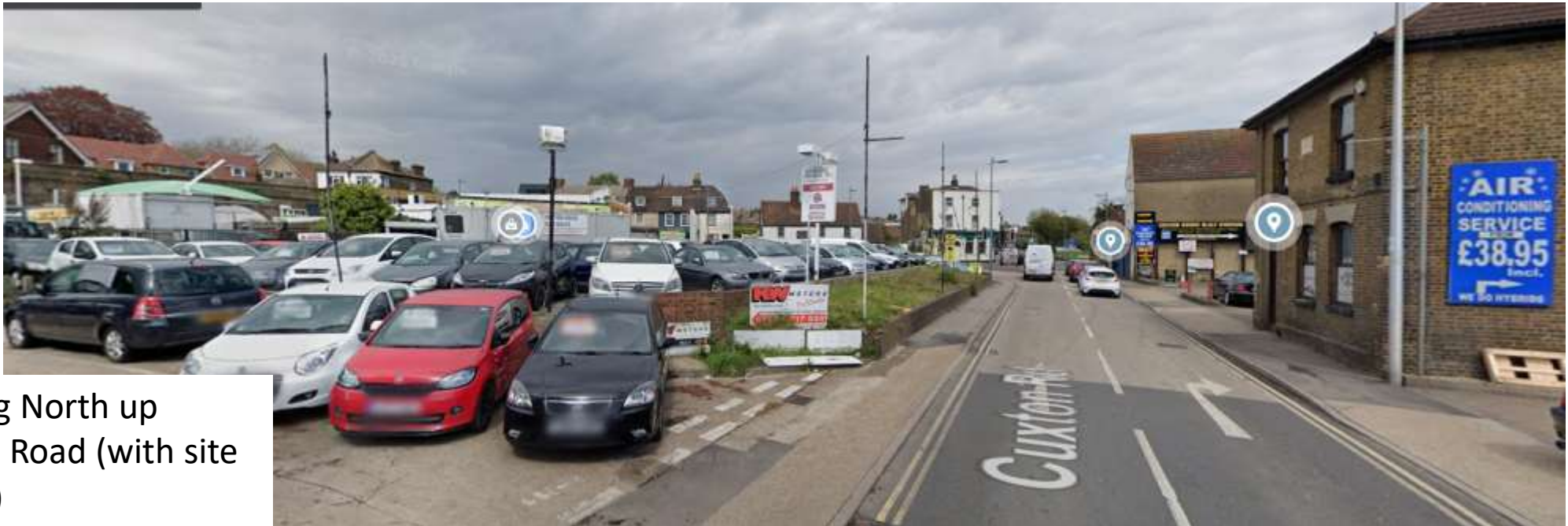
Looking east along London Road (from under railway bridge)
