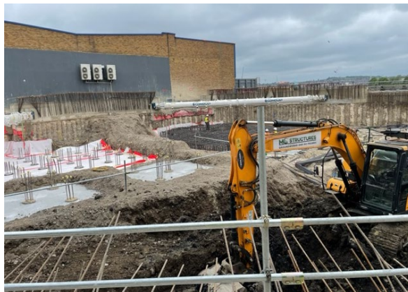
Photograph, showing podium car park excavation (Below Blocks A and E)
