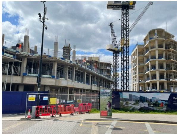
Photograph, showing concrete frames (Blocks B, C and D)
