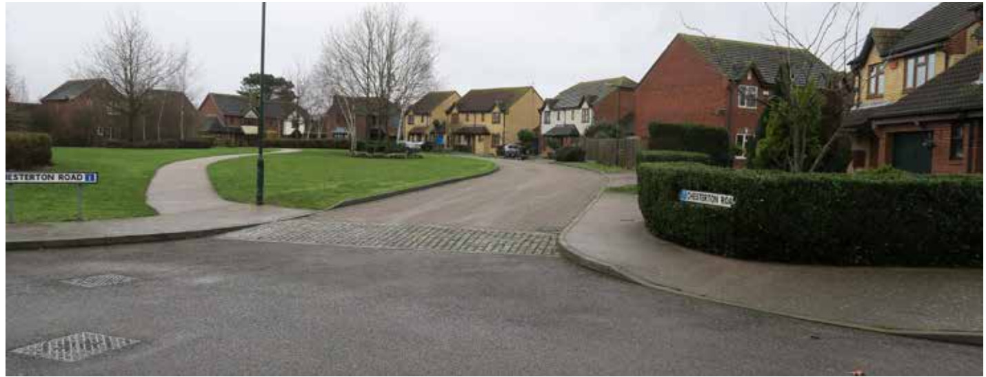
Figure 52: Shared area with block and sett surfacing on Chesterton Road. The well-kept landscaping and footpaths also encourage walking.
