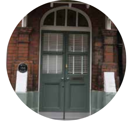
PAINTED DOOR FRAME
