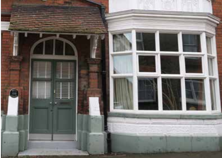
Red brick façade with painted door and window frames.
