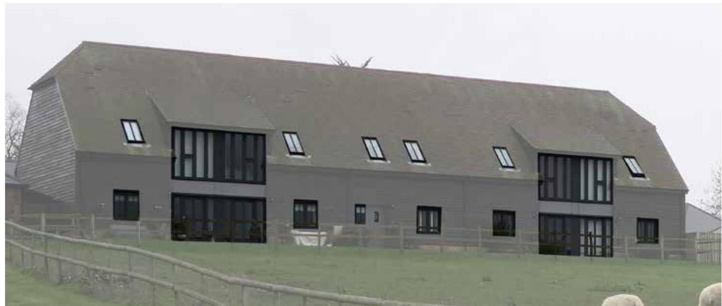
Figure 46: Contemporary building using variations in building rhythm and proportions to articulate the horizontal mass of the building
