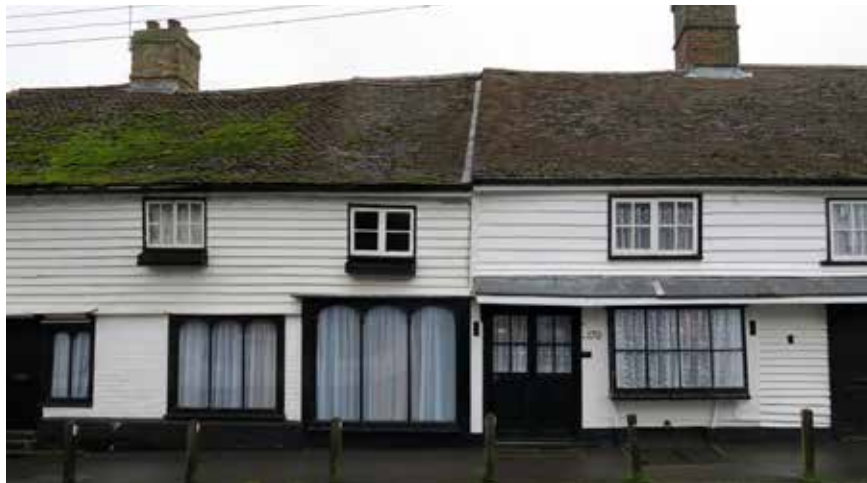
Figure 57: Grade II listed buildings with traditional white weatherboarding and clay roof tiles on Church Street.
