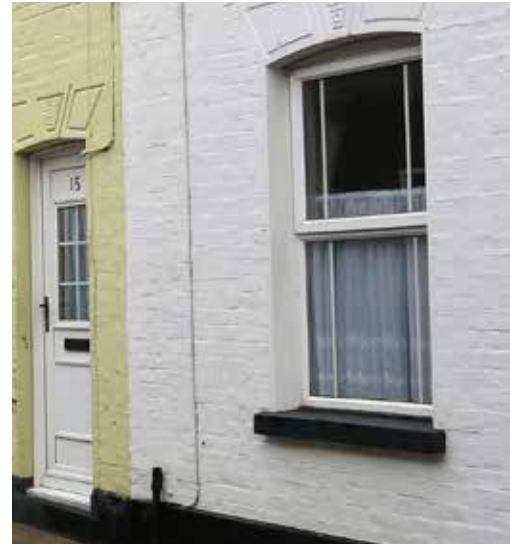
Victorian terrace houses with painted brick façades on Reed Street.
