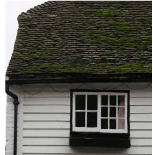
Listed building with a half-hipped roof with clay plain tiles and white weatherboarding.
