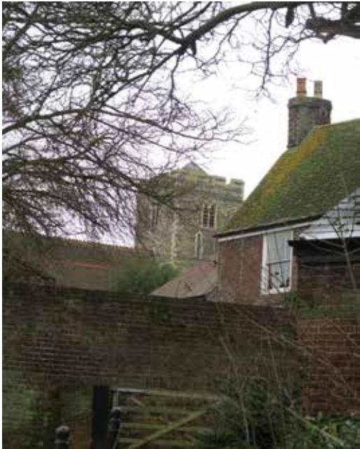
Figure 22: View of the Church of St Helen's clock tower from Pond Hill
