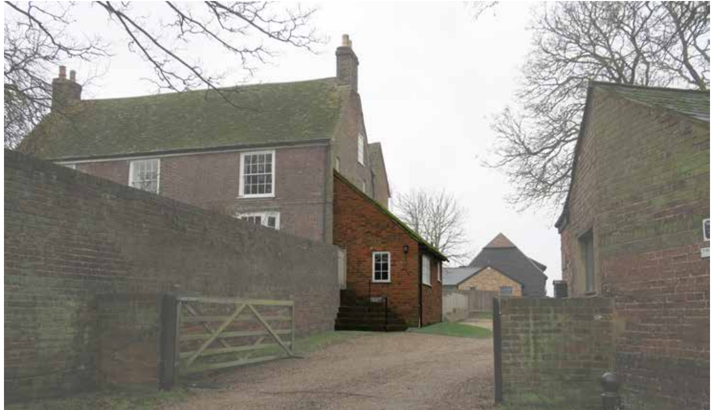
Figure 48: Successful side extension to a Grade II listed building.
