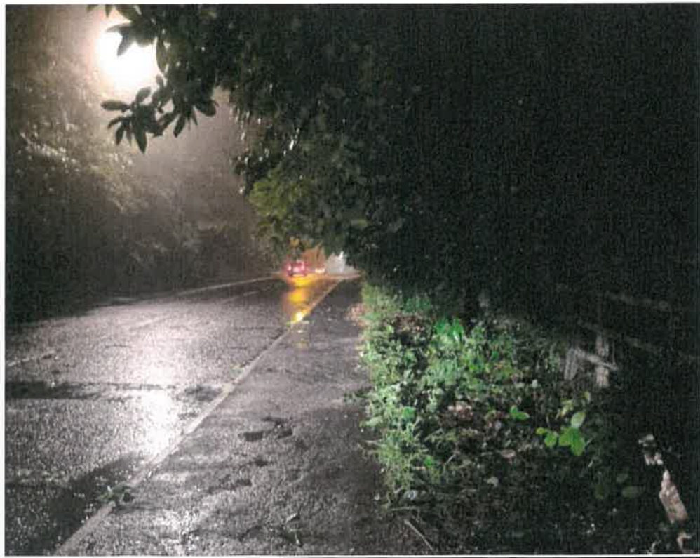
Callout, collapsed Tree leaning out towards Hoath Lane
