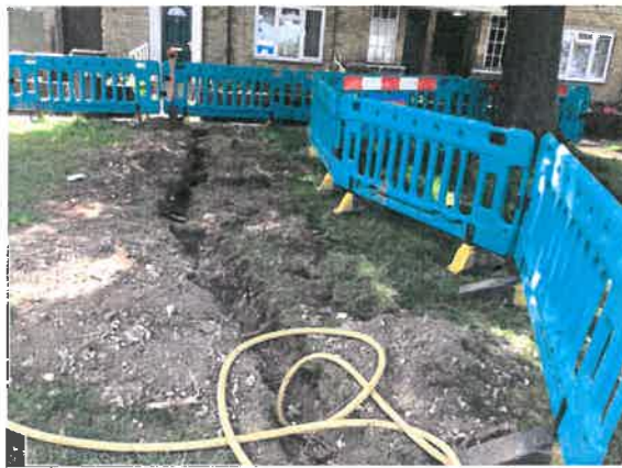
Careful trenching through a trees Precautionary Zone
