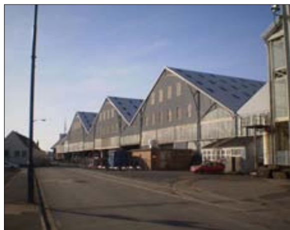
Covered Slip Buildings looking south
