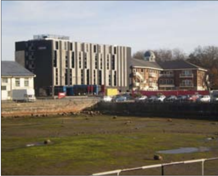
Existing view of the Lower Boat House, the Hotel and Office Block
