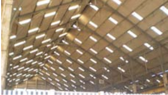
Roof structure inside the Covered Slip
