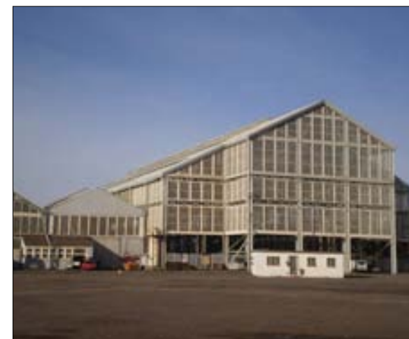
Photo showing the Covered Slip No. 7
