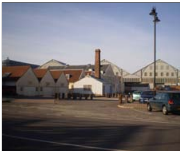
Photo showing Wheelright's Shop, the Old Forge and the Mould Loft in front of Covered Slips 4, 5 and 6.
