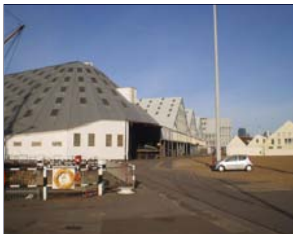
Covered Slip Buildings looking north
