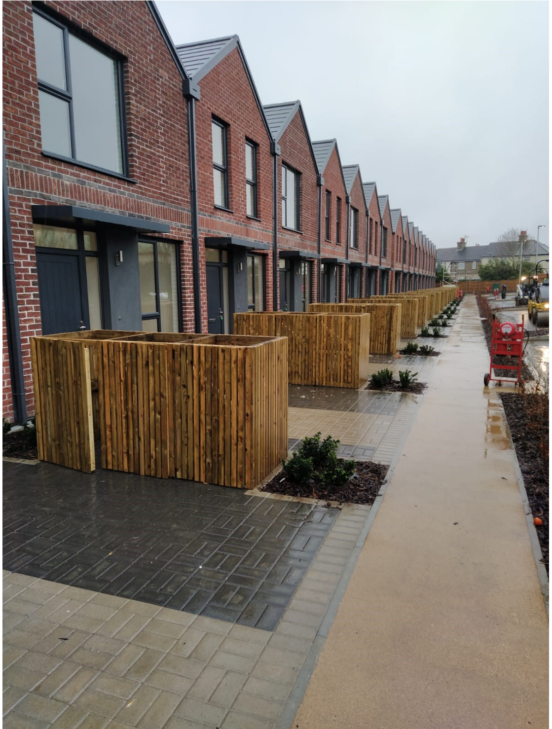
Fig 6. Photo of the completed White Road residential scheme January 2021.
