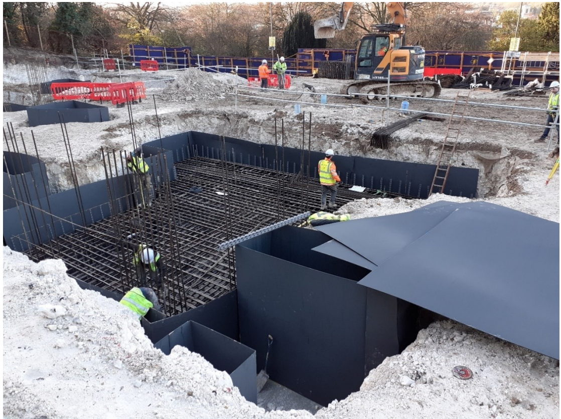
Fig5. Foundation works at Garrison Point January 2021.
