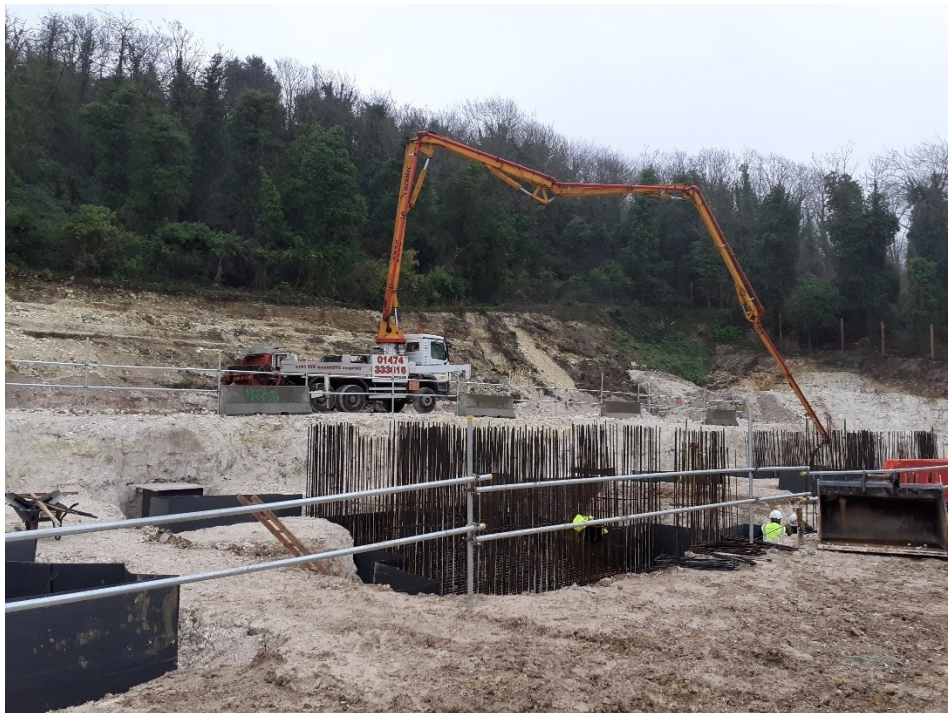
Fig4. Foundation works at Garrison Point January 2021.
