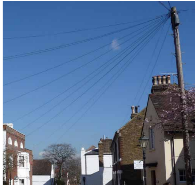
Surfeit of telephone wires
