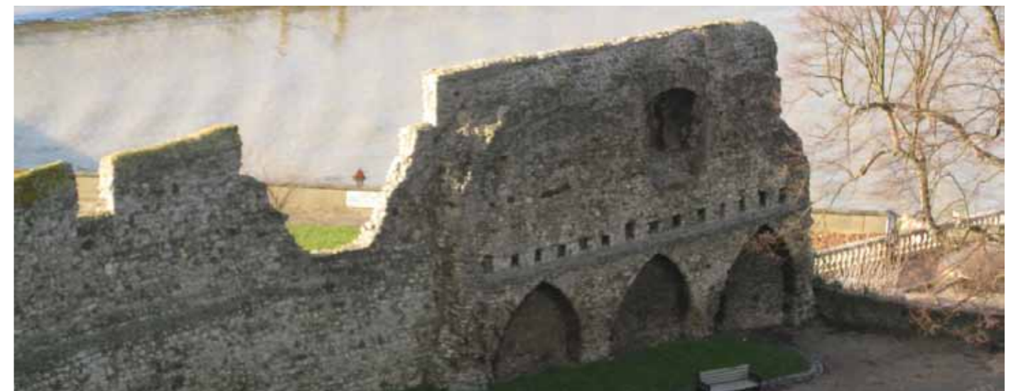
Section of Gundulph's curtain wall, the earliest surviving masonry
