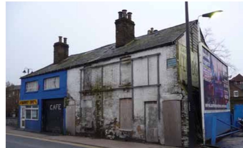
25-31 Corporation Street, buildings of little architectural merit
