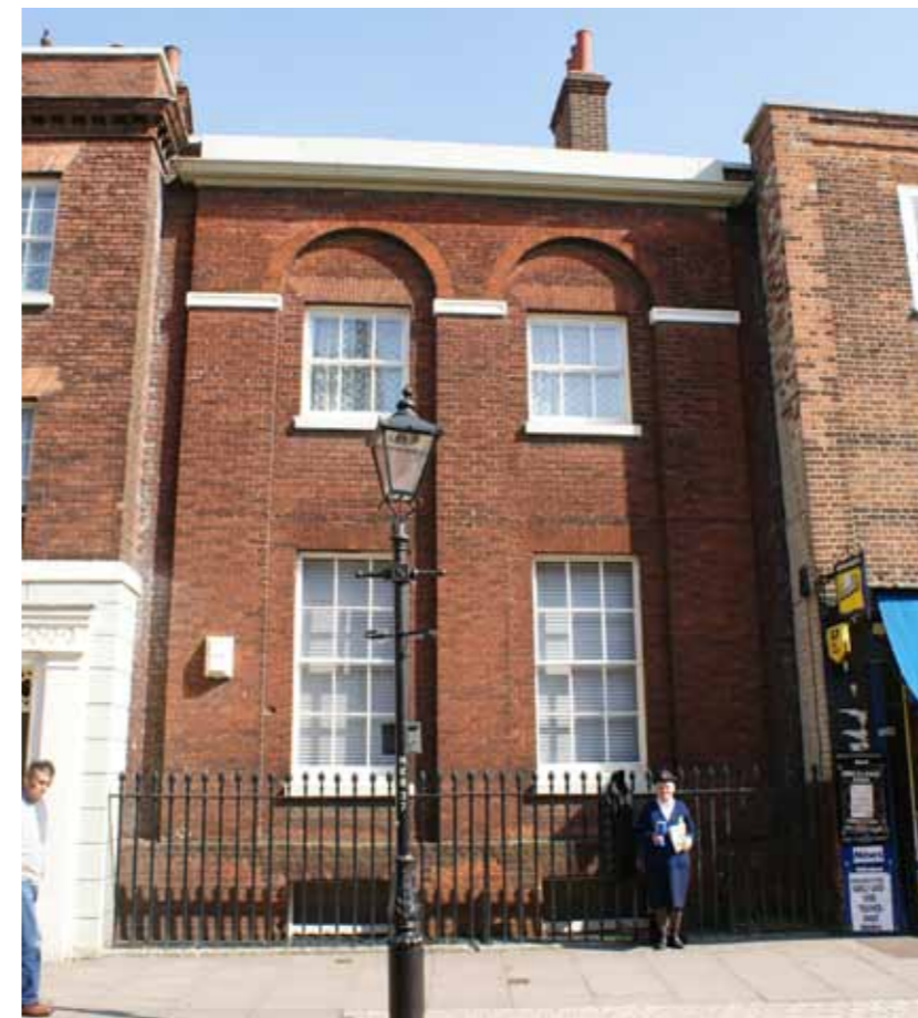
Example of a break in the building line at no. 109 High Street
