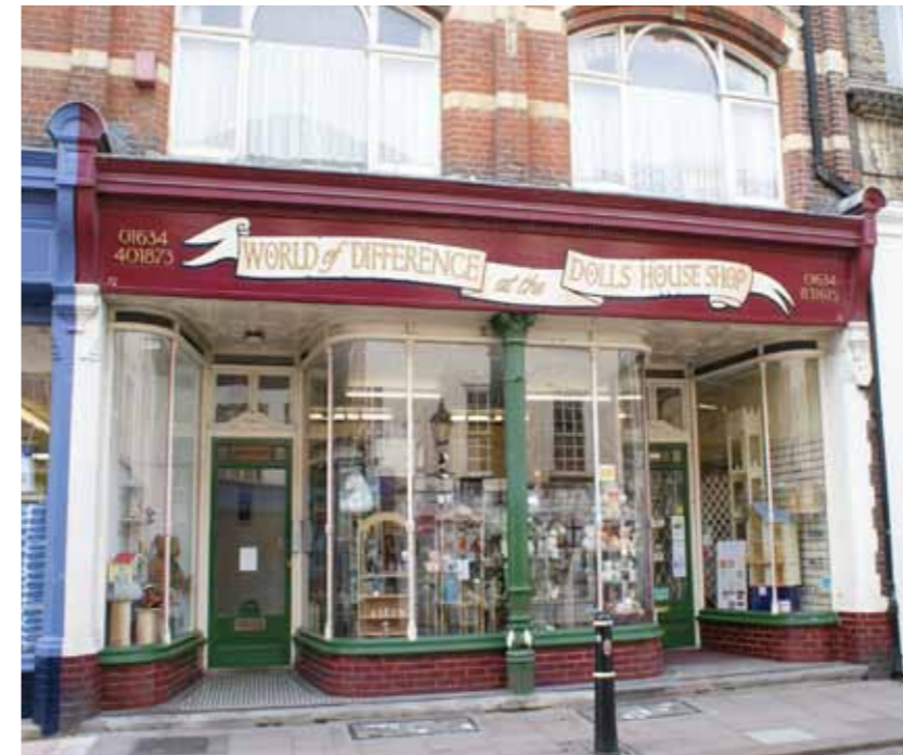
No. 72 High Street, a fine, distinctive Edwardian shopfront
