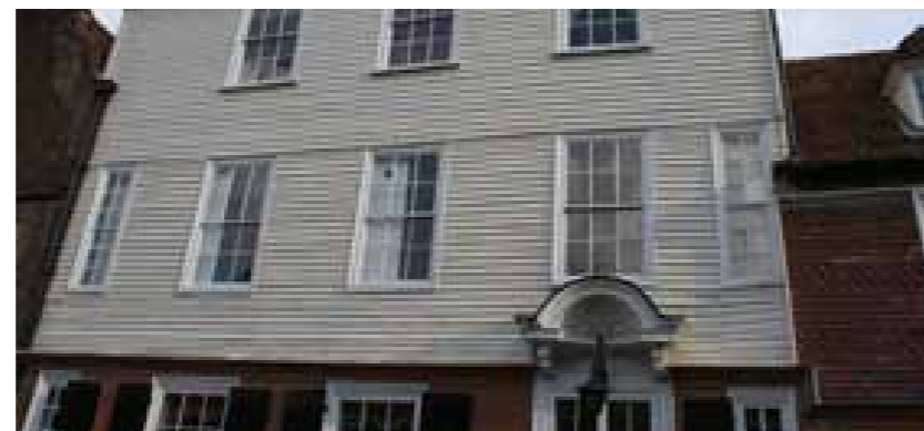
Vine House, timber cladding, a typical Kentish detail
