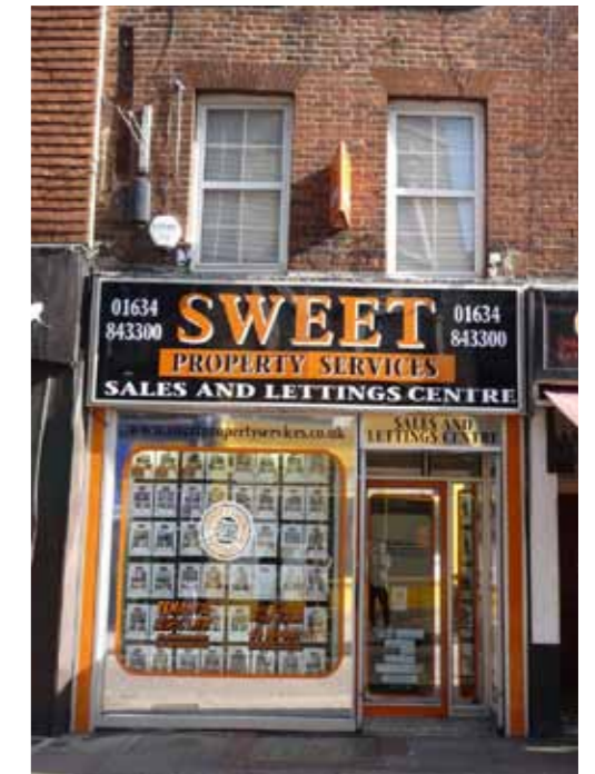
No. 175 High Street, removed stall-risers, UPVc fascia sign and metallic surround.
