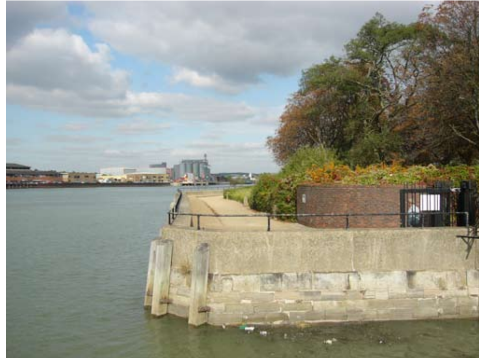
Gun Wharf Flood Defences
