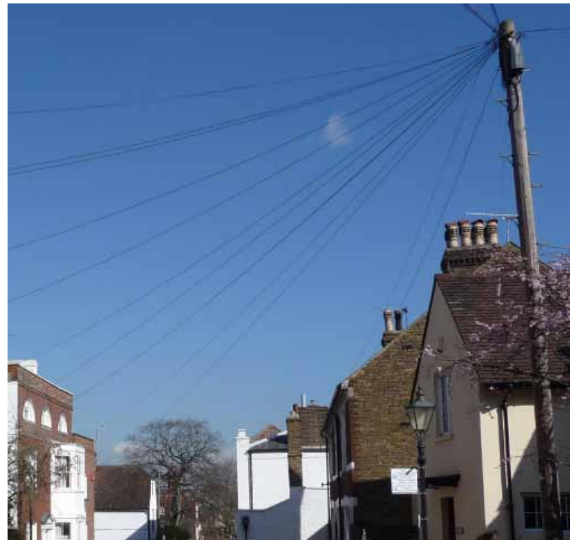
Surfeit of telephone wires
