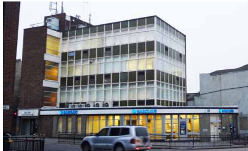
Barclay's Bank, a negative contribution to the conservation area
