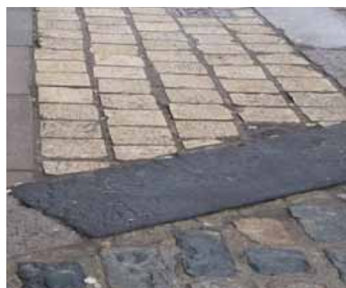
Varied paving materials on the High Street and side roads
