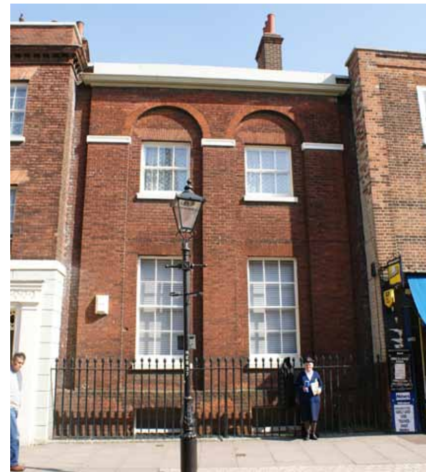
Example of a break in the building line at no. 109 High Street
