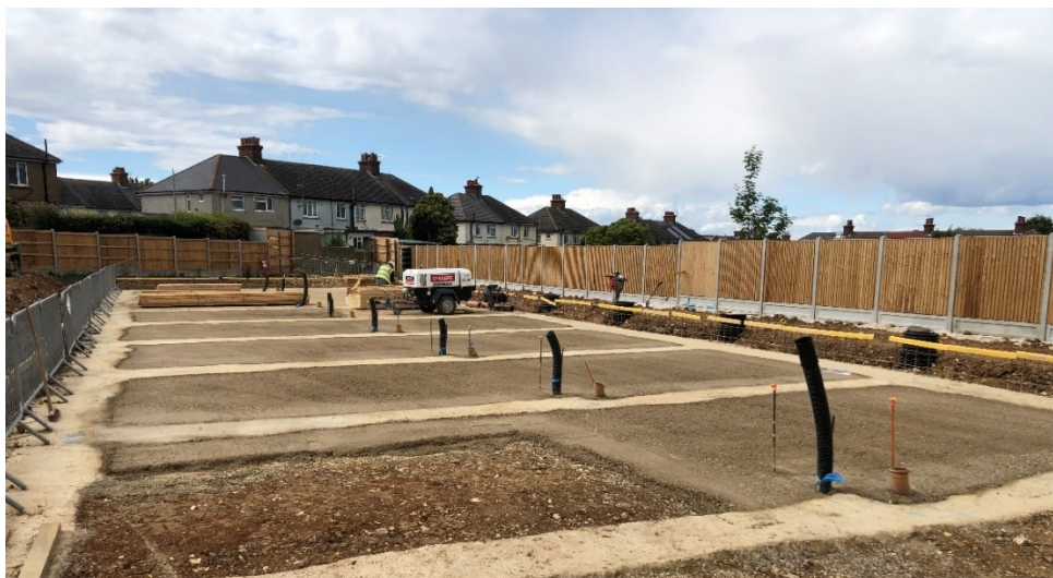
Fig5. Photo showing the preparatory ground works at the White Road site.
