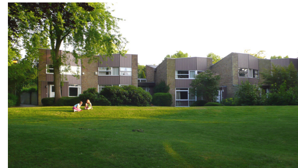
The Lane, Blackheath (above) and New Ash Green, Kent (below). 1960s housing designed by Eric Lyons for the Span Development Company.
