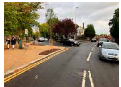
Chingford Lane in Walthamstow, where a road entrance has been narrowed to slow traffic and create public space Top image © Google
