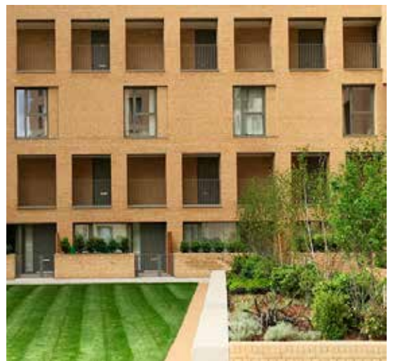
from left: Allies and Morrison, Hale Wharf Phase 2 Allies and Morrison, St Andrews Allies and Morrison, West Hendon
