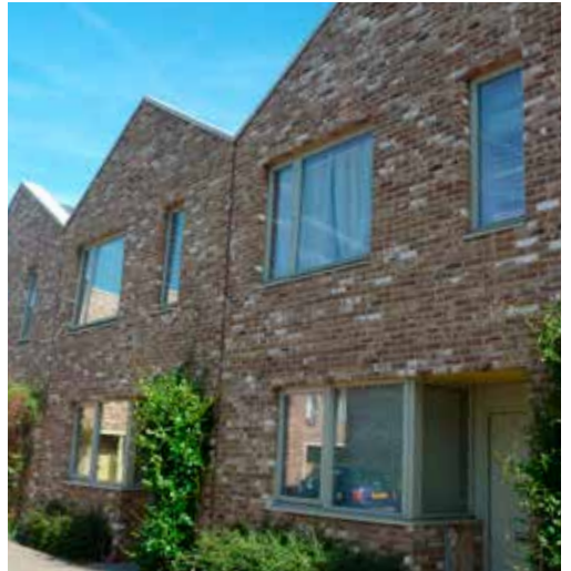
from left: FCB Studios, Accordia Housing, Cambridge ©Sebastian Ballard / Wikimedia Commons Barking Riverside AHMM and MaccreanorLavington Architects, Anne Mews, Barking
