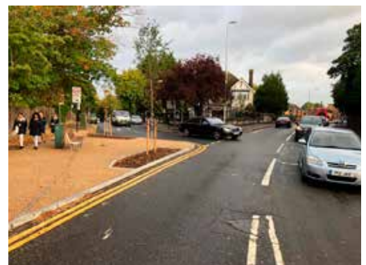
Chingford Lane in Walthamstow, where the road entrance has been narrowed, encouraging traffic to continue ahead or take the turning very slowly. Top image © Google
