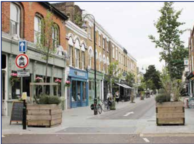
Orford Road was dominated by vehicular traffic with a poor urban environment and narrow footways, frequently blocked by parked coaches, cars, and street clutter. The new development introduced public realm improvements, with the road narrowed to allow only for local buses with restrictions for vehicles and motorcycles from 10am to 10pm.
