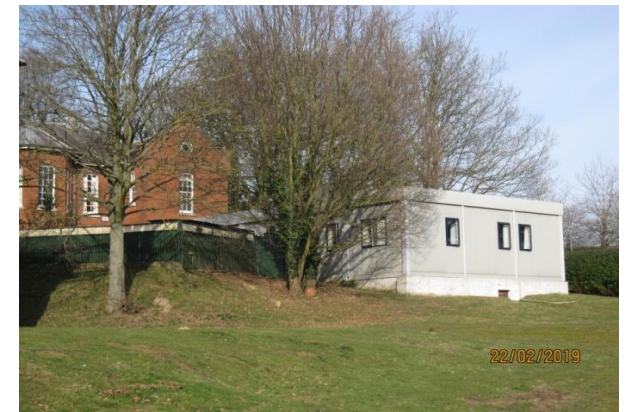
Cranmer Temporary extension
