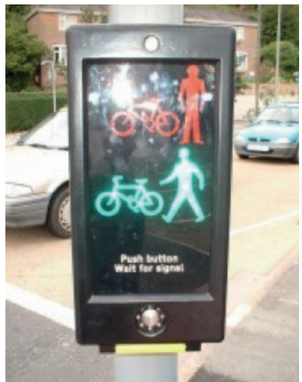
Figure 2: Toucan crossing display box to support cyclists
