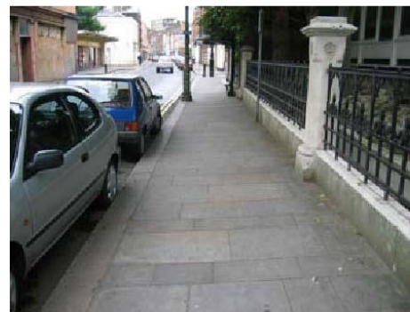
Reinstated yorkstone paving
