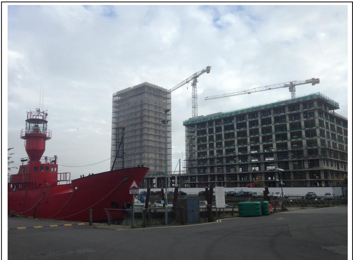
LV21 lightship and development at Victory Pier, Gillingham
