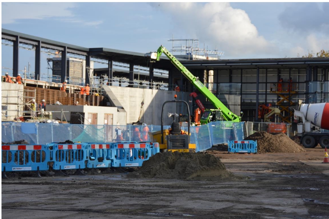
Construction of new Rochester railway station Photo by Jamie Ives
