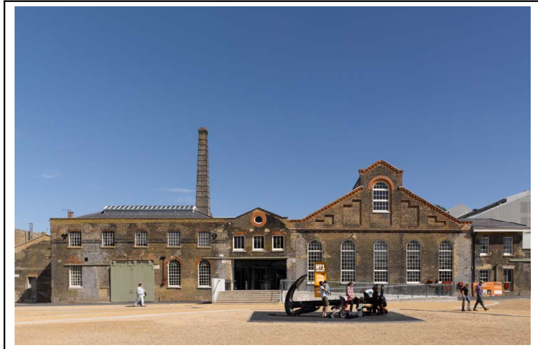
No 1 Smithery – Chatham Dockyard
