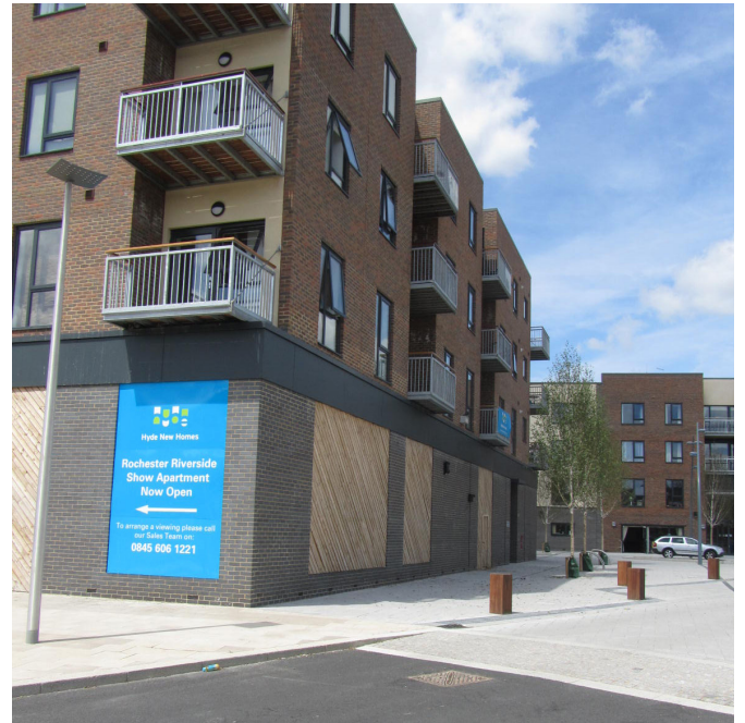
First phase of development completed in 2013
