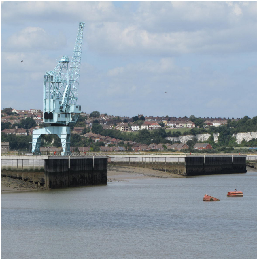
Existing Blue Boar Wharf
