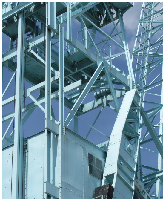
Distinctive crane at Blue Boar Wharf
