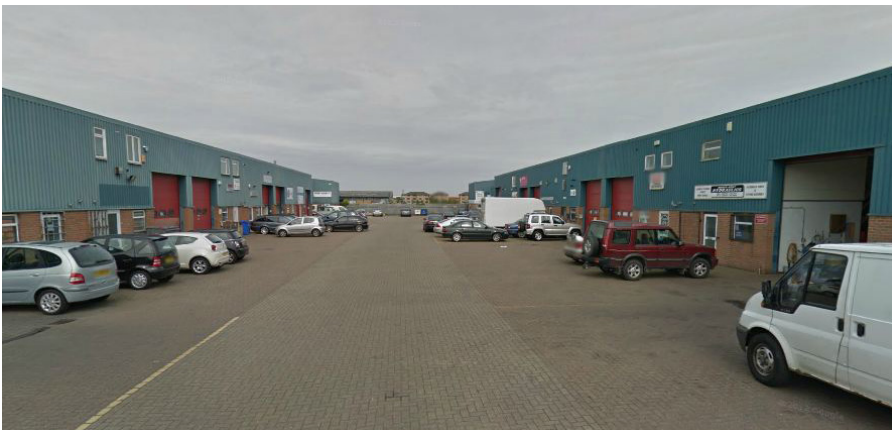
Existing Castle View business park
