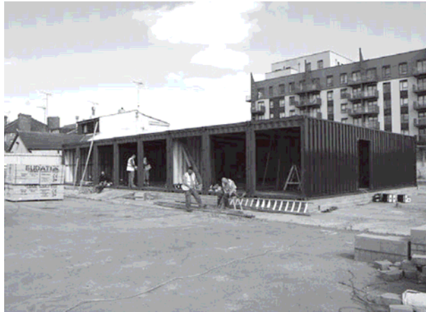
Construction of the accommodation at the depot
