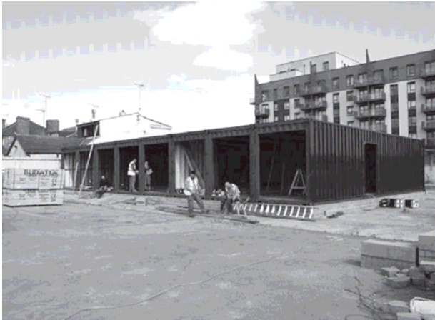
Construction of the accommodation at the depot
