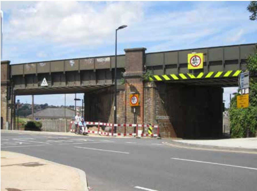
Gas House Road junction
