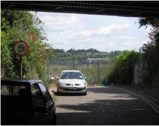
View under the railway to the site
