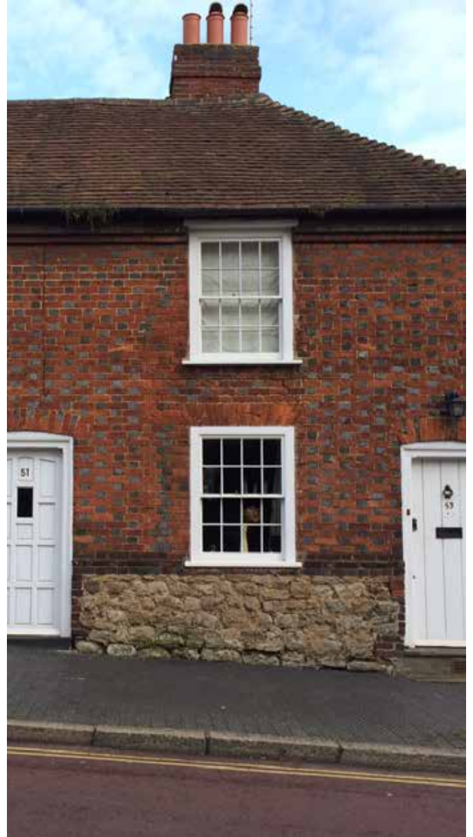
Combination of natural stone, decorative brick and slate roof tiles
