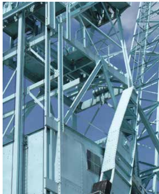
Distinctive crane at Blue Boar Wharf
