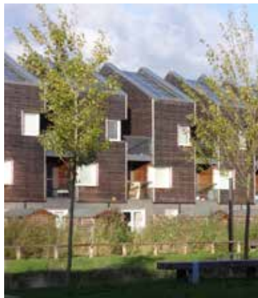
Terraces, Barking Riverside
