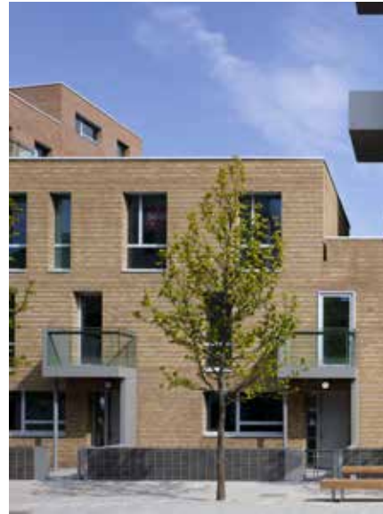
Balcony elements form an integral part of facade design
