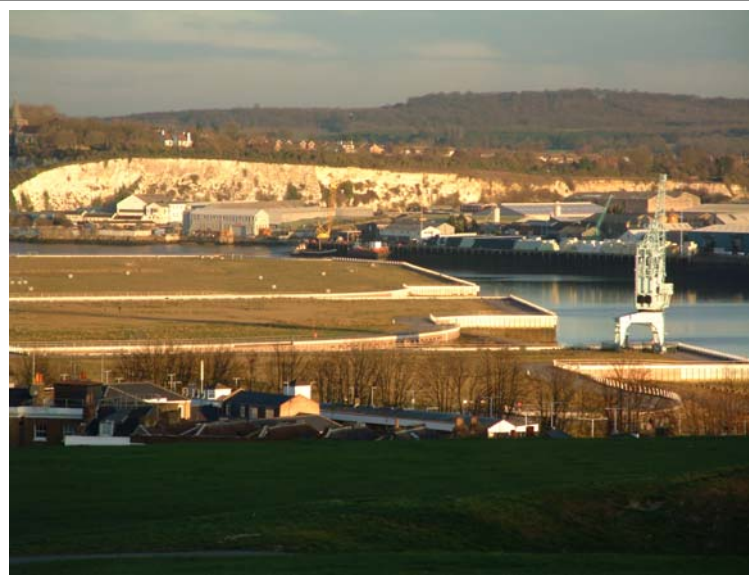
Flood defences at Rochester Riverside
