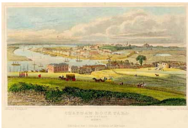
Roffe 1829 'Chatham Dockyard from Fort Pitt'. (c) Medway Archives. Note Barrier Ditch and openness of landscape of Lines.
