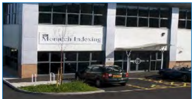
Figure 5.14: A Whilst the majority of car parking should be to the rear of buildings, it is helpful to locate a small amount of visitor and disabled parking at the front, along with cycle parking for visitors.
