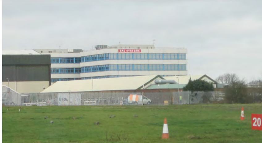
The draft core strategy states: "BAE Systems is by some way the area's largest private sector employer and the company is a global leader in its field. The company itself has identified opportunities for spin-off activities and land is available to develop complementary employment facilities. This could create an economic 'cluster' of considerable significance."
