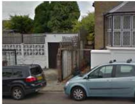
Existing Boundary Conditions
