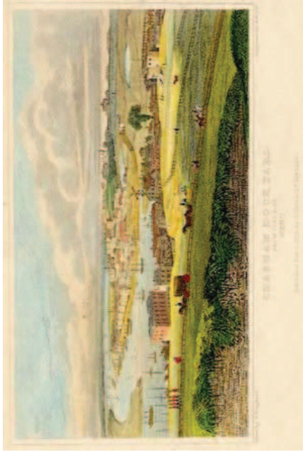
Roffe 1829 'Chatham Dockyard from Fort Pitt'. (c) Medway Archives. Note Barrier Ditch and openness of landscape of Lines.
